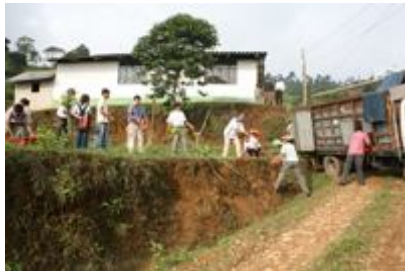
Unloading construction materials
